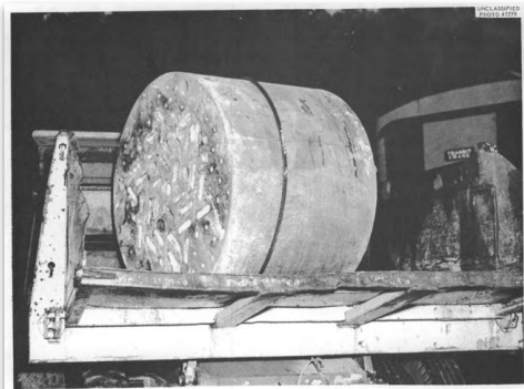
Fig. 23. Bottom View of Reactor Ready for Transfer to Burial Ground.
