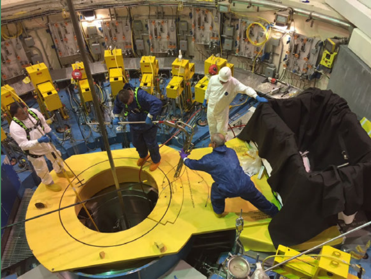
Segment Pipe Cutting and Removal
