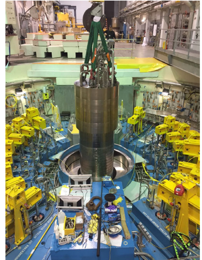
IRP-2 Being Lowered into Core Vessel
