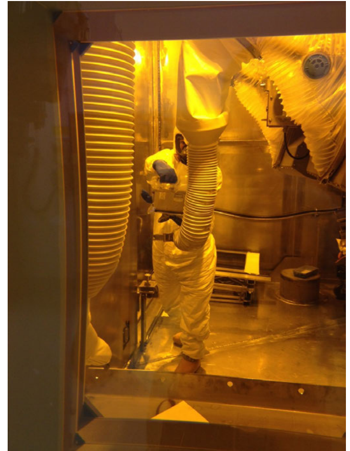
Radiation Control Technician surveying servo grips during Transfer Bay entry
