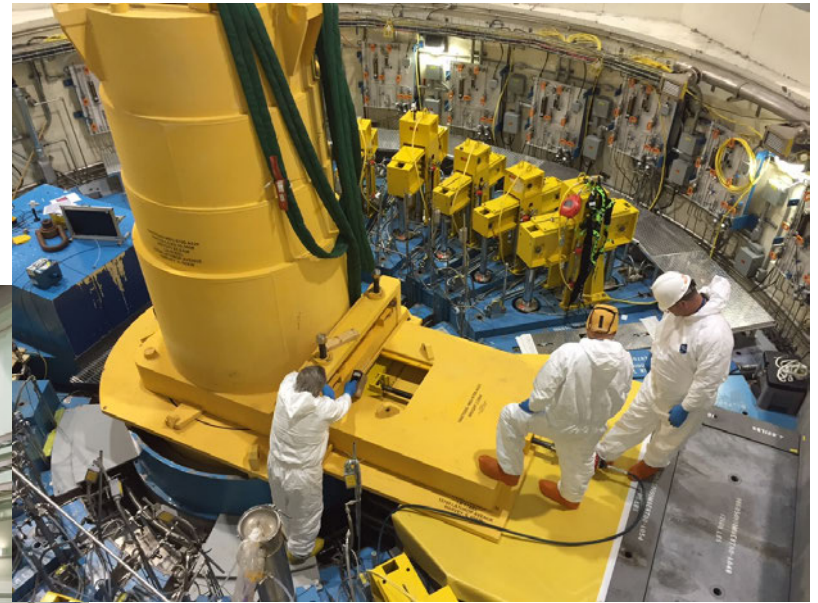
Installation and Testing of Shielded Door Assembly
