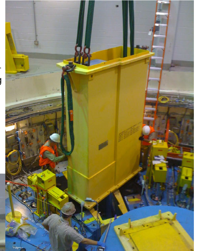
Removal of Upper Shutter Plug
