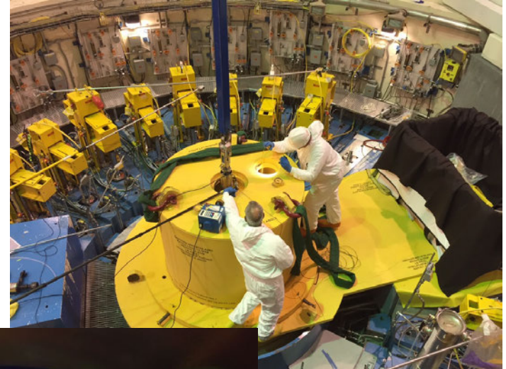
Pulling Segment up into Cask
