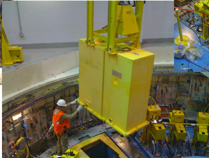
Installation of Shielded Cask for Lower Shutter Plug Removal
